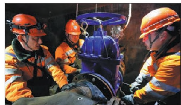
Pipeline workers of Jixi Hydropower Section replace a leaking valve in the main water supply pipeline.
