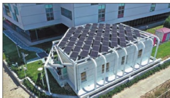
Top: The Fourth Community of the China-Singapore Tianjin Eco-City on Sept 27, 16 years after the project's beginning in 2008. LI RAN / XINHUA Above: The "zero energy emissions and zero carbon" building in the eco-city. PROVIDED TO CHINA DAILY
