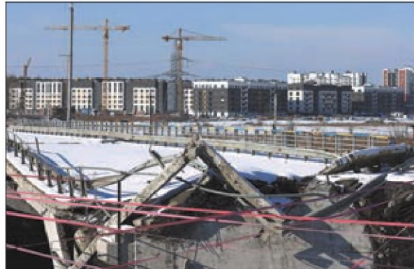
A bridge destroyed to prevent Russian troops from advancing is seen in Irpin, Ukraine, on Tuesday. THE YOMIURI SHIMBUN VIA AP IMAGES
