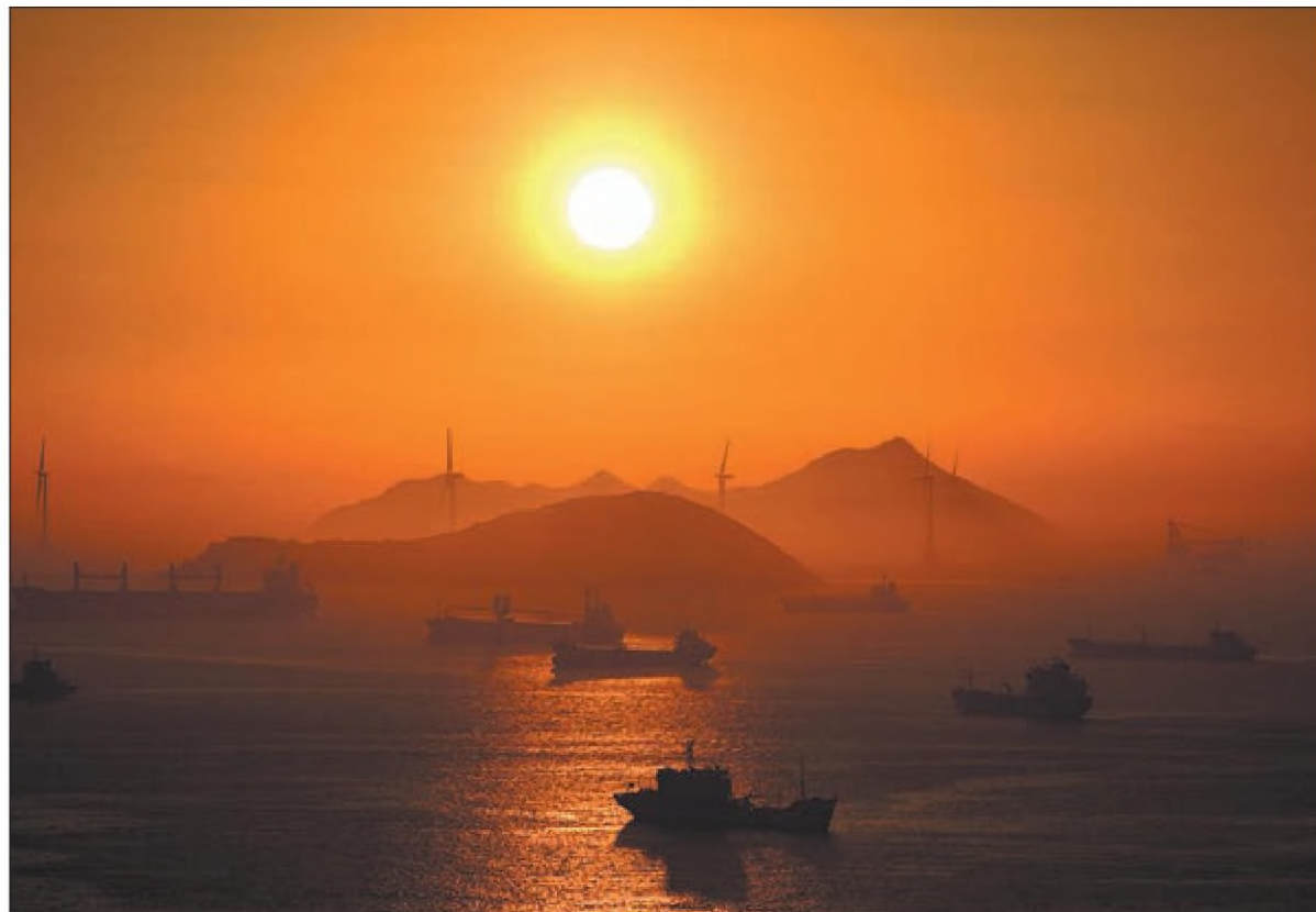
An image shows an offshore wind farm in Guangdong province. As of the third quarter of 2024, a total of 39.1 million kilowatts of offshore wind power capacity in China had been connected to the grid. ZHOU GUOQIANG / FOR CHINA DAILY
