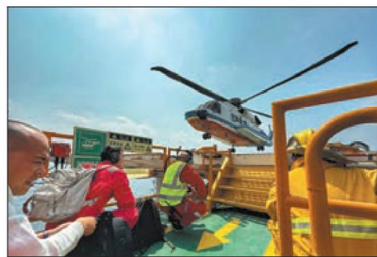
A helicopter lands on a massive deck of the Enping 15-1 offshore oil production platform.
