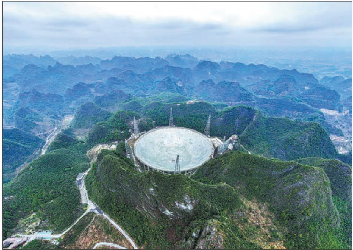
An aerial photo of the Five-hundred-meter Aperture Spherical Radio Telescope (FAST) project situated in mountains in Pingtang county, Guizhou province, in February last year. OU DONGQU / XINHUA
