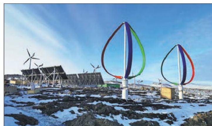
The water-drop-shaped devices are the latest wind turbine developed by Taiyuan University of Technology, which feature effective resistance to low temperatures and strong winds. PROVIDED BY TAIYUAN UNIVERSITY OF TECHNOLOGY
