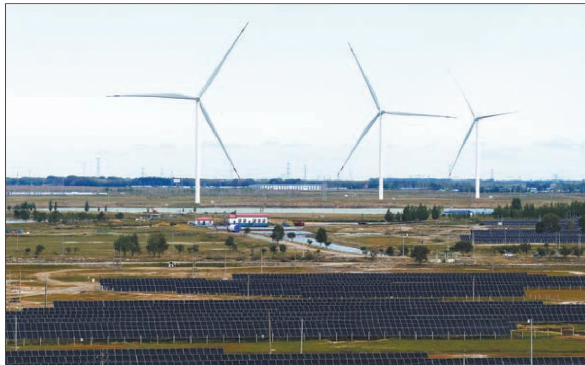
An image shows a solar and wind power station in Daqing, Heilongjiang province, in September. The station is part of Daqing Oilfield's efforts to ramp up green transition and achieve decarbonization goals. YANG WEI / XINHUA
