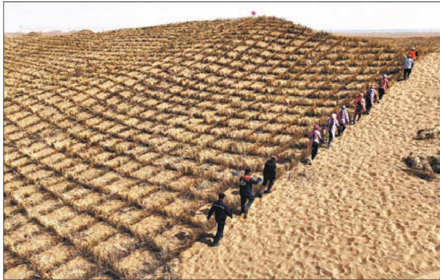
Workers plant grass grids at a sand control site that is part of the Three-North Shelterbelt Forest Program in Gaotai county in Zhangye, Gansu province, on Tuesday. Gaotai is located on the southern edge of the Badain Jaran Desert, China's third-largest desert. This year, the county plans to set green barriers on 1,800 hectares of sandy areas. CHENG LIN / FOR CHINA DAILY
