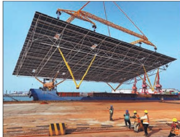
Left: A crane lifts a large steel photovoltaic platform onto a ship in Laizhou, Shandong province, on Feb 27. TANG KE / FOR CHINA DAILY
