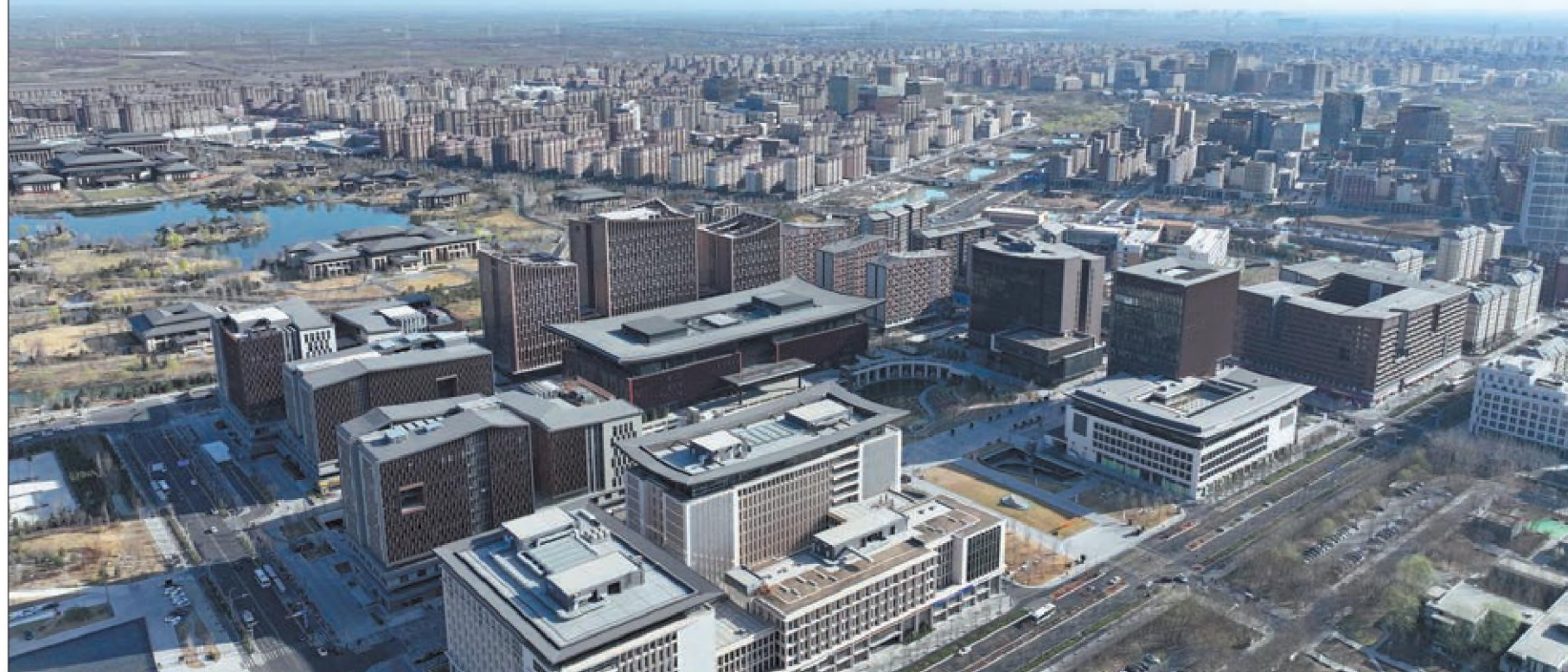
An aerial photo of the Xiong'an Business Service Center and Rongdong area in Xiong'an New Area, Hebei province, taken on March 21. PHOTOS BY WANG JING / CHINA DAILY
