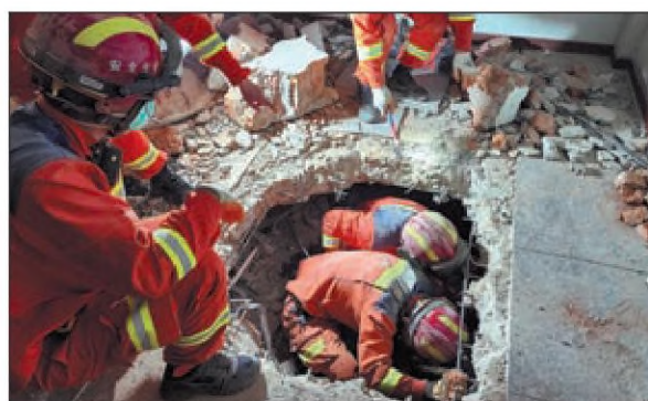
China's Yunnan rescue and medical team works at the ruins of Odalatli Hospital in Nay Pyi Daw, Myanmar, on Sunday. WANG CHANGHUA / FOR CHINA DAILY
