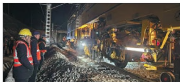
Workers from China Railway Taiyuan Bureau Group realign tracks on the 347-kilometer Datong-Taiyuan Railway as part of work to ensure safe transport across the network. JI XIAOQIANG / FOR CHINA DAILY
