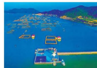
Xiangshan's Huangbi'ao township uses environmentally friendly composite materials for fishing pontoons. PROVIDED TO CHINA DAILY
