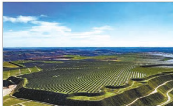
Photovoltaic panels are installed on a reclaimed area of Changxu coal mine in Narisong, Inner Mongolia autonomous region, in August. The project uses green solar energy in the process of making hydrogen. PROVIDED TO CHINA DAILY
