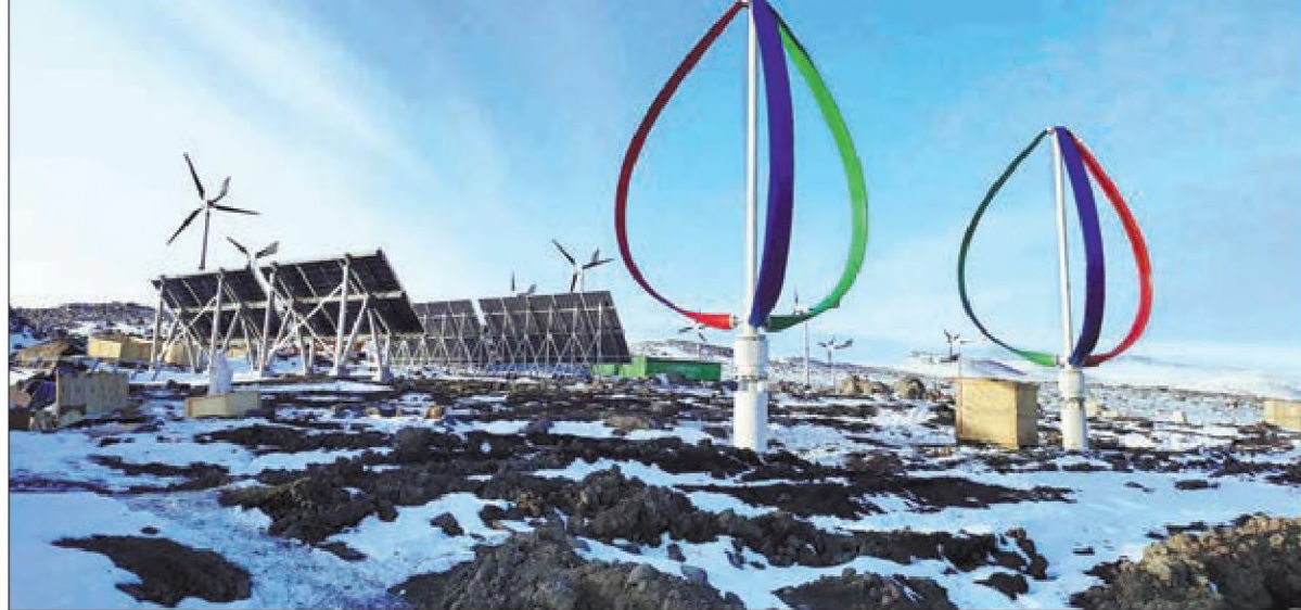
Two droplet-shaped wind turbines spin in front of China's Qinling station in Antarctica. PROVIDED TO CHINA DAILY
