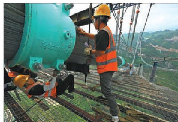
Workers operate on the Huajiang Grand Canyon Bridge in Guizhou province on Sept 11, 2024. LEI SHENG / FOR CHINA DAILY
