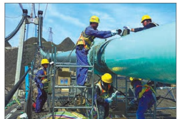
Workers cooperate on the nearly completed Huajiang Grand Canyon Bridge in Guizhou province on April 21, 2025. ZHANG JIE / FOR CHINA DAILY
