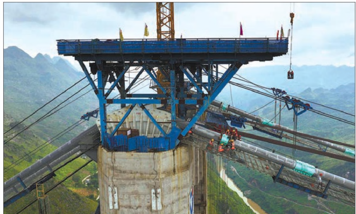
A photo shows the Huajiang Grand Canyon Bridge under construction in Guizhou province on Sept 11, 2024. LEI SHENG / FOR CHINA DAILY
