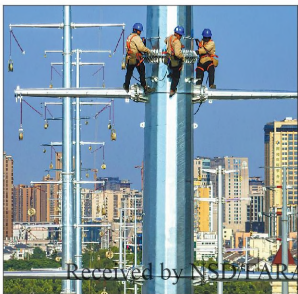
Technicians from State Grid Suqian Power Supply Co install power lines for a 220-kilovolt power transmission project in Suqian, Jiangsu province — a project to elevate the city's peak summer load. Once operational, it will help eliminate the only medium and long-term Level 5 risk in Suqian's power grid, guaranteeing the grid's stable operation. WU DI / FOR CHINA DAILY
