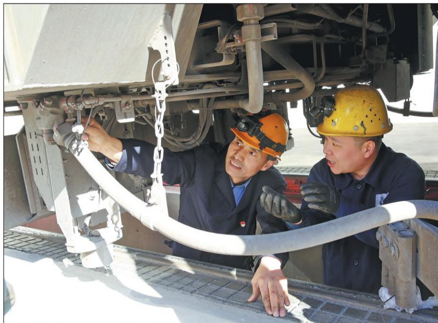
Technicians from the Houma North Locomotive Depot of China Railway Taiyuan Group Co Ltd conduct maintenance checks on braking systems, sanding devices, wipers, lighting and high-voltage equipment, in order to safeguard railway transportation during the upcoming rainy season.
