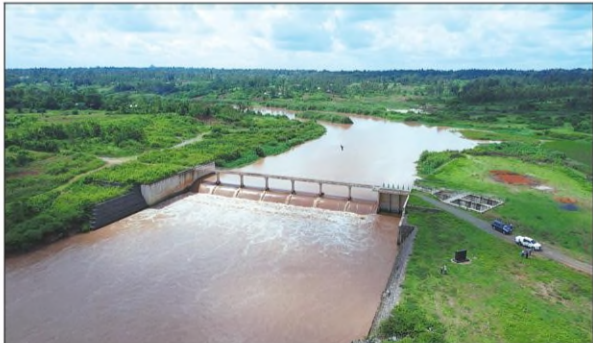
An aerial view of the head works of the Chinese-built Lower Nzoia Irrigation Project. WANG YUXI / CHINA DAILY
