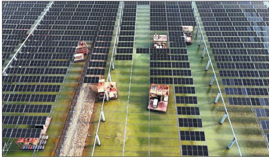
Technicians install solar panels at a saltern in Lianyungang, Jiangsu province. GENG YUHE / FOR CHINA DAILY
