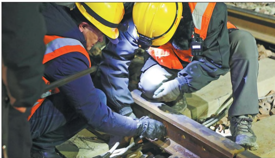
The Yuanping Track Division of China Railway Taiyuan Group Co Ltd recently launched a 15-day concentrated maintenance operation on the 355-kilometer Datong-Taiyuan railway line in Shanxi province. By upgrading 167 kilometers of tracks along the route, they will improve safety and reliability for passengers and cargo. Over 600 employees are taking part in the project. YANG HONGXING / FOR CHINA DAILY
