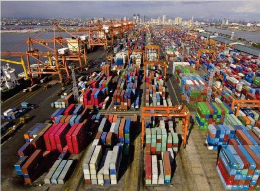
Honduran President Juan Orlando Hernández applauded the progress of a new 396-kilometer national highway, known as the "Dry Canal," connecting the Atlantic port of Puerto Cortés with the Pacific ports of Amapala and Henecán on the Gulf of Fonseca.
