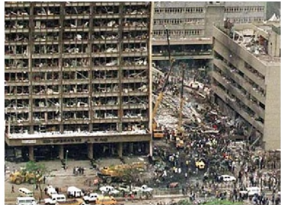
All photos in this section courtesy of Partners New York Times
