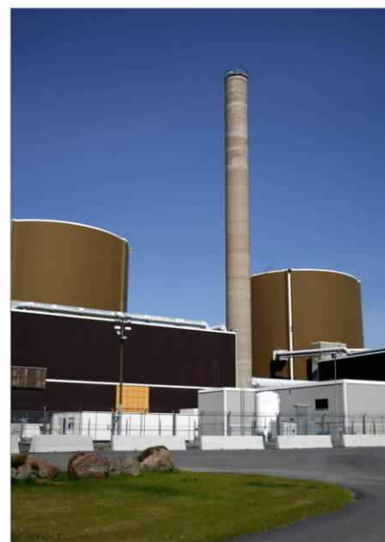
Fortum's pilot Power-to-X plant will be built next to an existing nuclear plant in Loviisa, Southern Finland. CREDIT: Fortum
