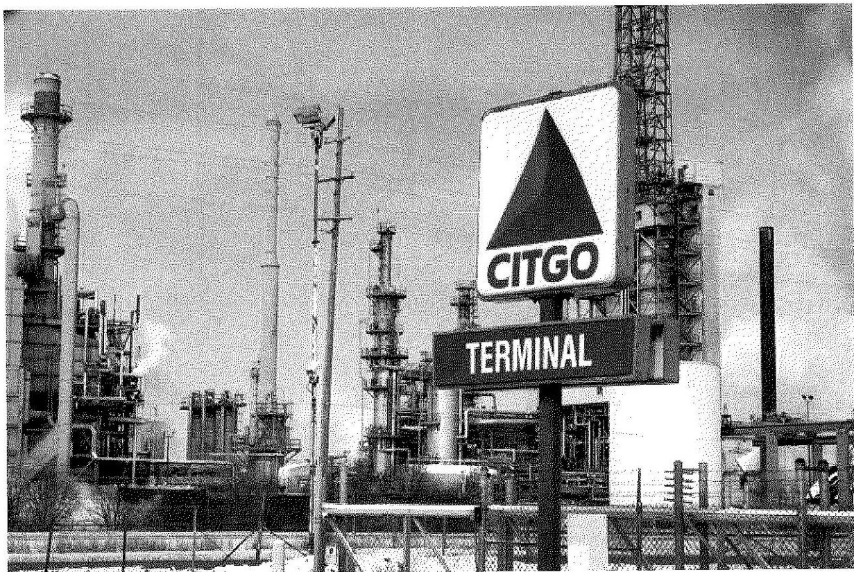
LEMONT, ILLINOIS - FEBRUARY 01: Smoke rises from a refinery owned by Citgo, a subsidiary of PDVSA, ...
