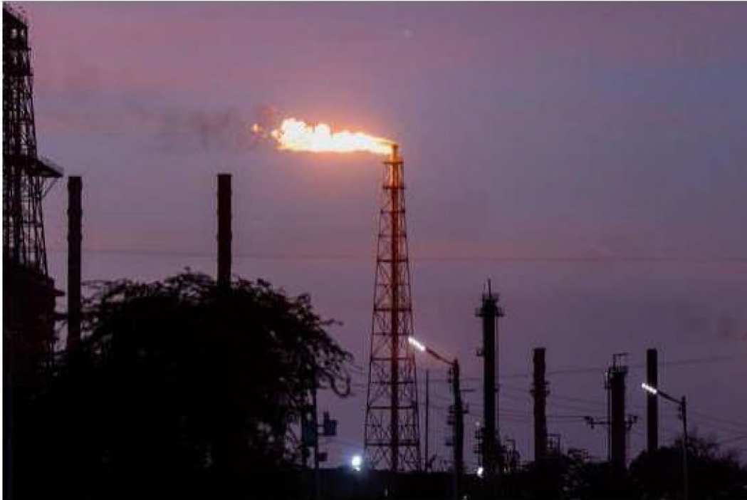
PDVSA Refinery Complex in Punto Fijo, Falcon State, Venezuela. Photographer: Betty Laura Zapata/Bloomberg
