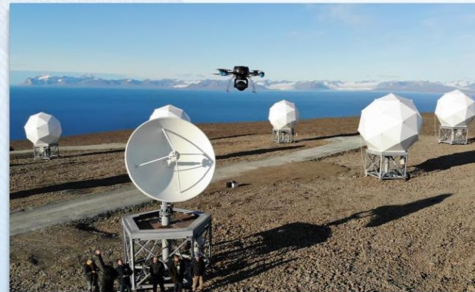
OneWeb – Svalbard and Nuuk teleports 3.7 m XY – Ku band. Subreflector alignment and calibration.
