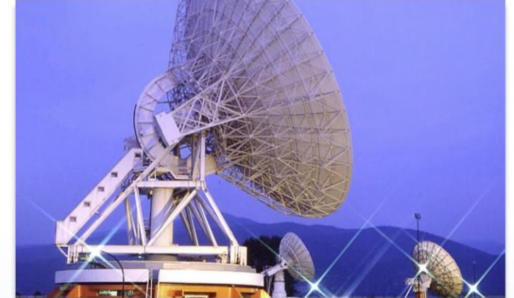
TELESPAZIO – Italy, Fucino Teleport 17m earth station – Ka band Validation after frequency upgrade.
