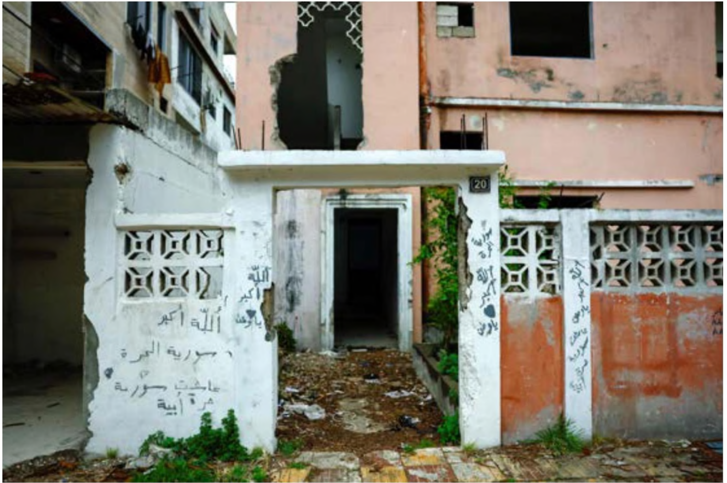
A damaged Alawite house in the Syrian city of Jableh, with graffiti reading: "God is Great," "Syria is free" and "long live Syria." The neighborhood came under heavy attack in March, when nearly 1,500 Alawites were killed by pro-government forces. The deaths marked a turning point for the two men plotting uprisings from exile. REUTERS/Stringer
