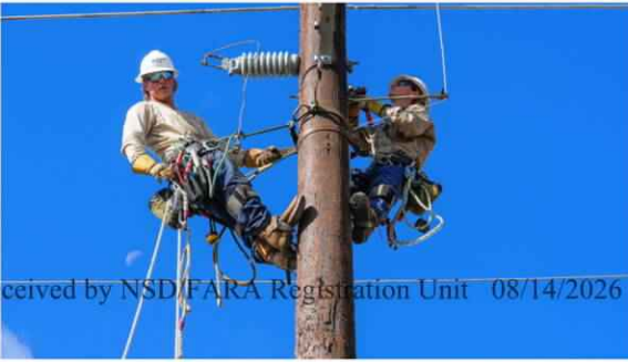
Apprentice linemen train in transformer bank construction at CenterPoint's Hiram O. Clarke Training Center in Houston on Wednesday, Nov. 12, 2025. (Raquel Natalicchio/Houston Chronicle/Getty Images)
