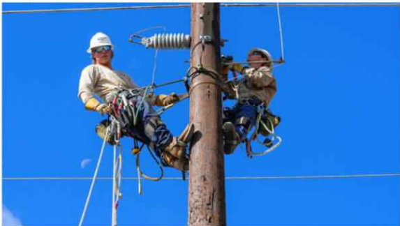
Apprentice linemen train in transformer bank construction at CenterPoint's Hiram O. Clarke Training Center in Houston, Wednesday, Nov. 12, 2025. (Raquel Natalicchio/Houston Chronicle/Getty Images)
